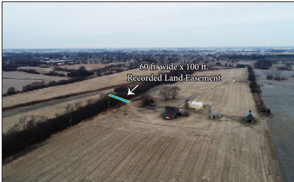
Aerial view of building site
