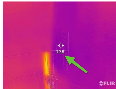
Heating temperature reading at return
