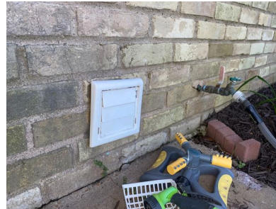
Dryer exhaust termination
