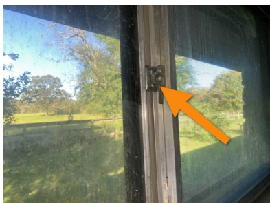
Window latch will not engage
