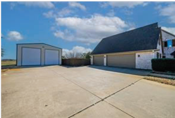
WORKSHOP...33x42, Two 12x14 Overhead Doors And One 10x8 Door Plus Walk-Thru Door, 220 Electric, 30AMP RV Connection And A 3 Car Oversized Garage Large Enough For Dually Or Boat
