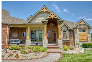
Front Of Structure
