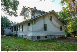
Side Of Structure
