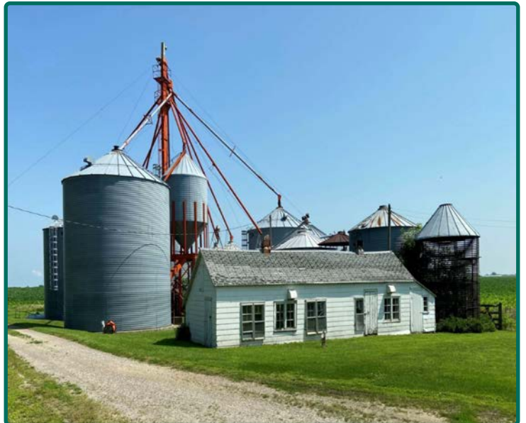
Grain Storage Area
