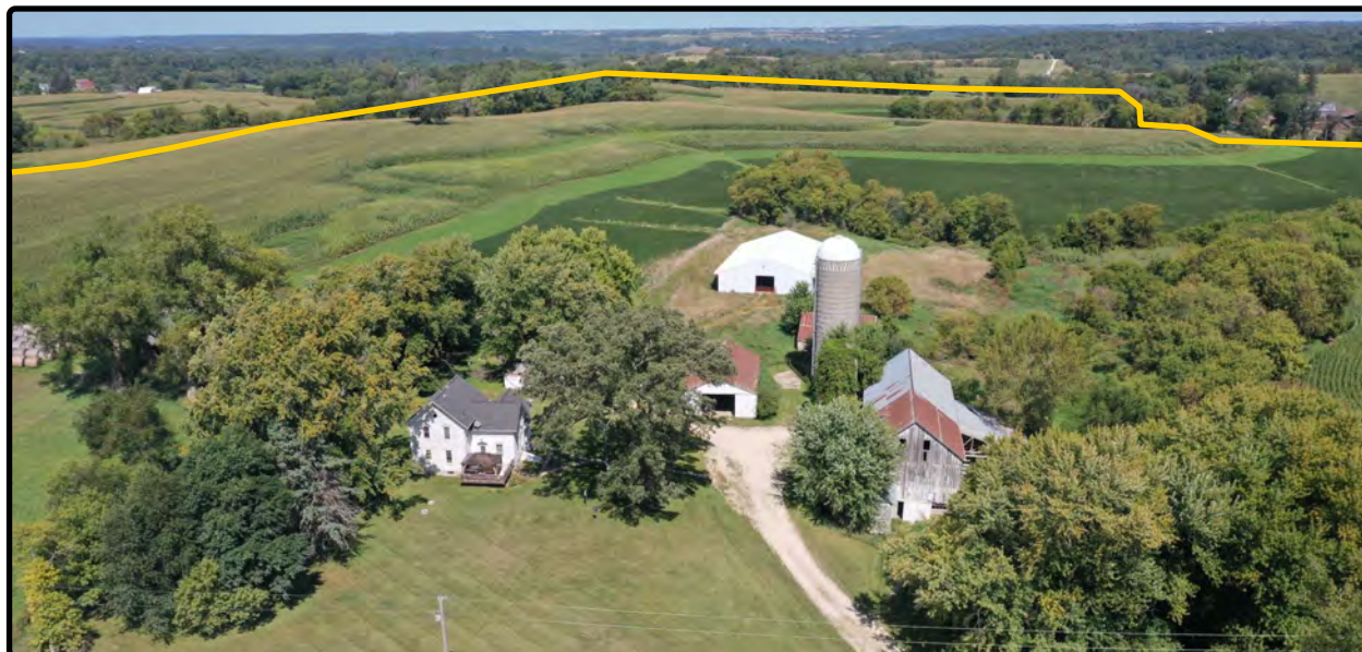
Parcel 1 - Building Site
