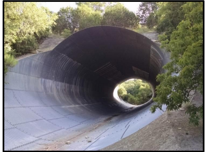
Culvert in Devil's Holland under FM 306 Courtesy of Paula Rieker, 2017
