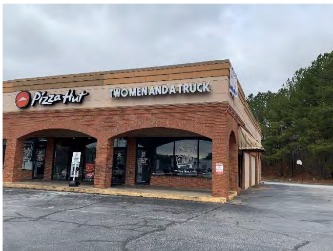
Potential offsite drycleaner
