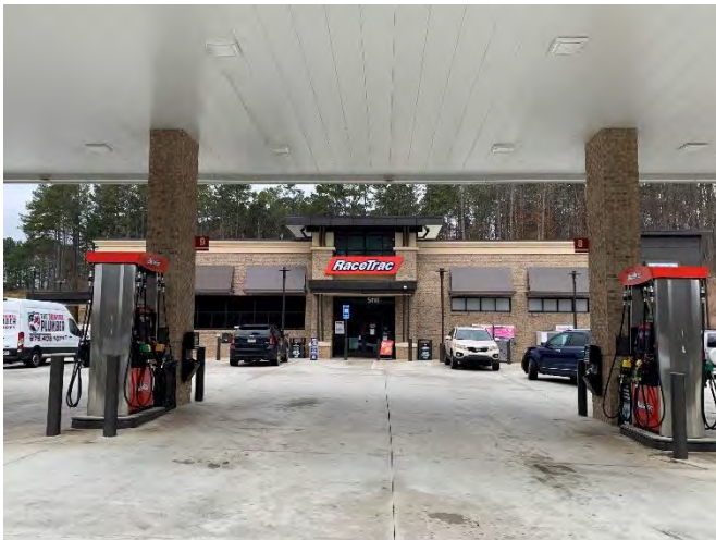
Offsite gas station
