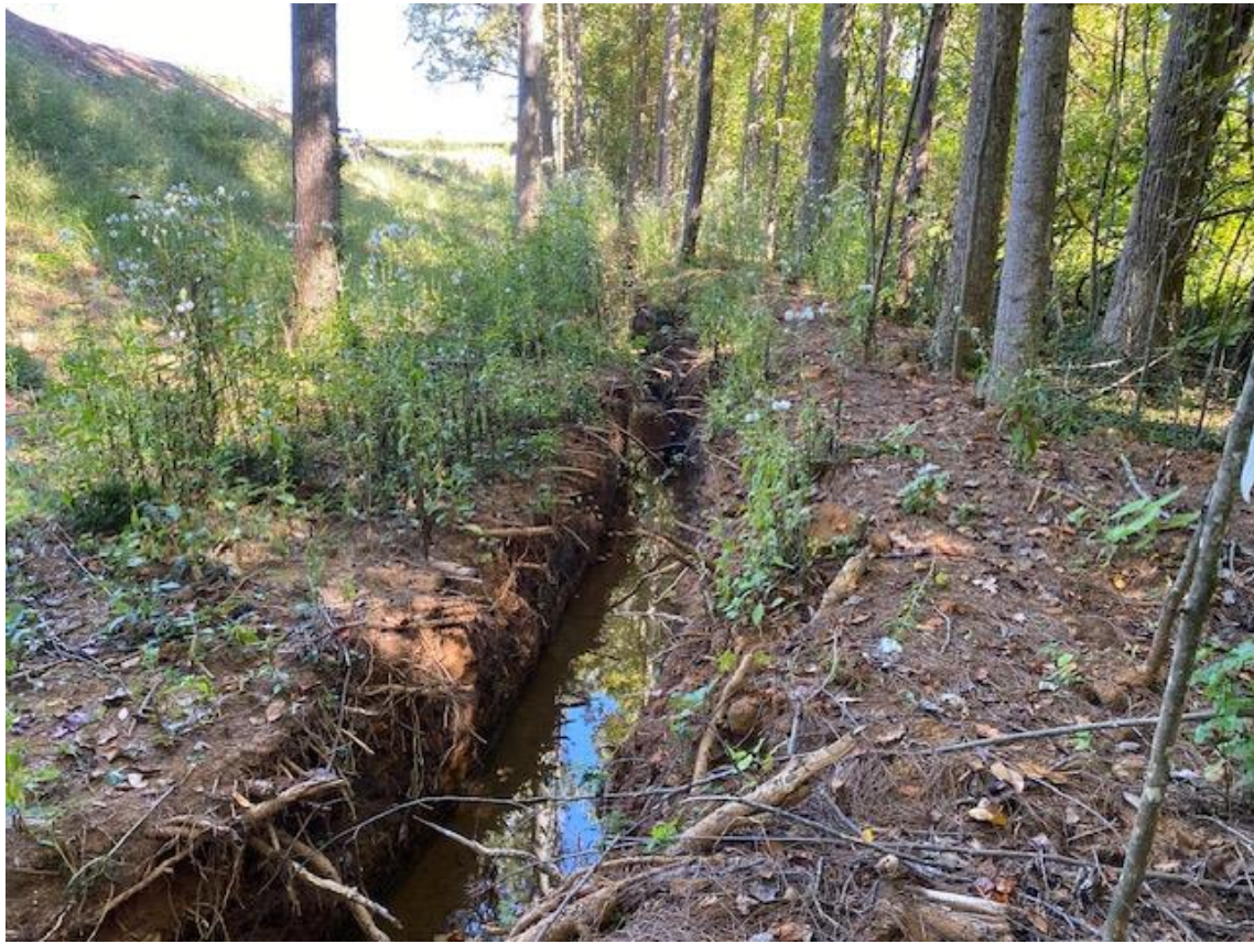
Photo 11: Photo of the recently excavated intermittent ditch located along the west of the site boundary.
