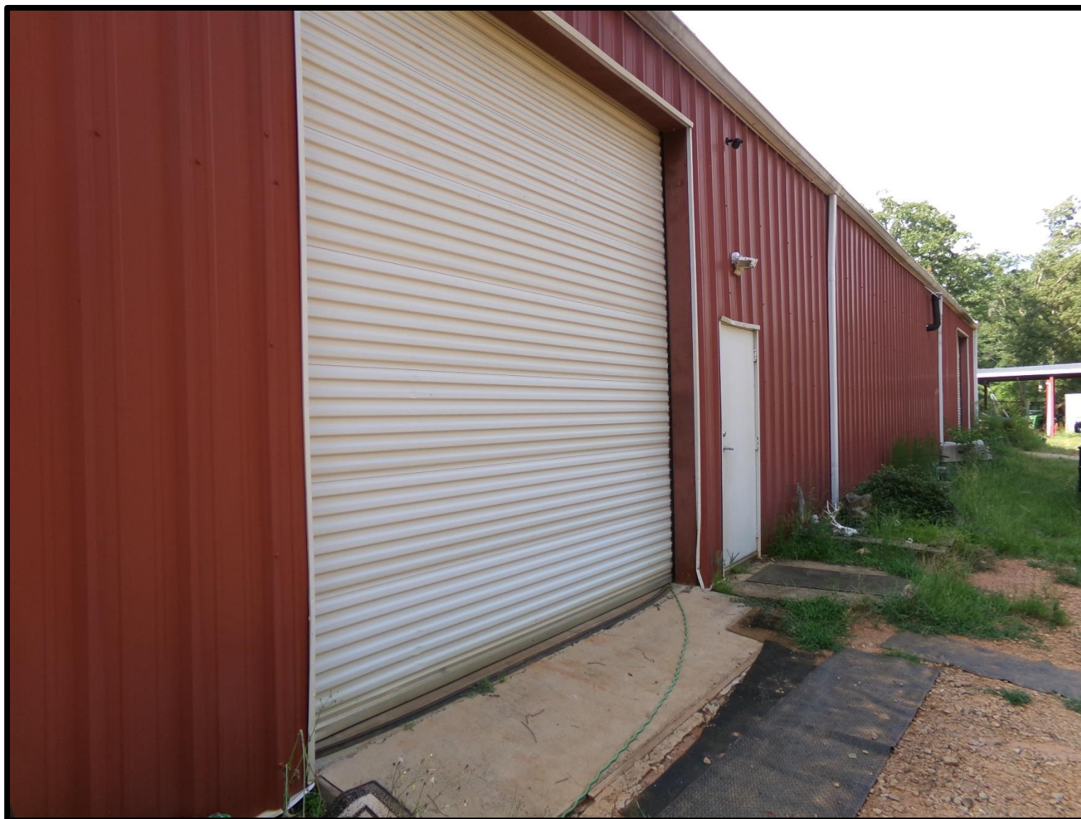
PHOTO 17, SHOP BUILDING Kevin Witcher (770-778-7188) Jackson Realty
