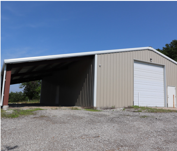
East Face of Building
