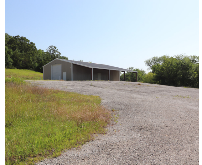
2,400 Sq Ft Metal Building + 1,200 Sq Ft Awning
