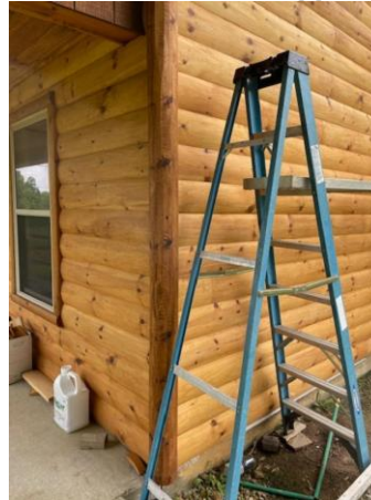
Cabin Siding Application
