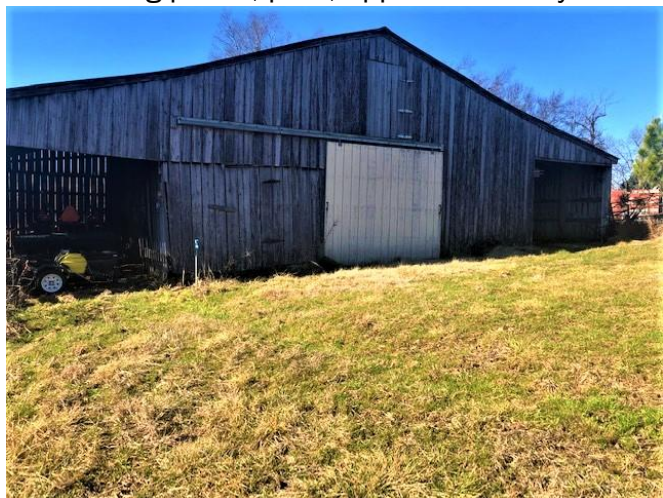
Existing Barn will hold equipment and ATV/UTV's
