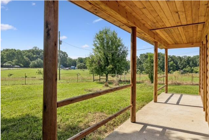
Porch columns, rails and ceiling
