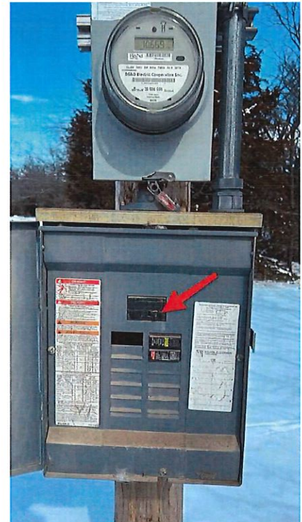
Exterior Service Panel: Panel Amperage 100 Amps
