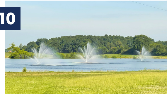
COMMERCIAL FOUNTAINS (4) 5 HP, 250' CORDS | (1) 1 HP, 100' CORD (INSTALLED 2022-2023)
