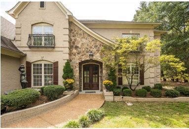
Front Of Structure
