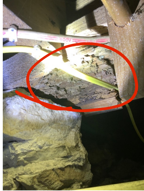
Both pictures crawl space opening beam over opening termite damage.
