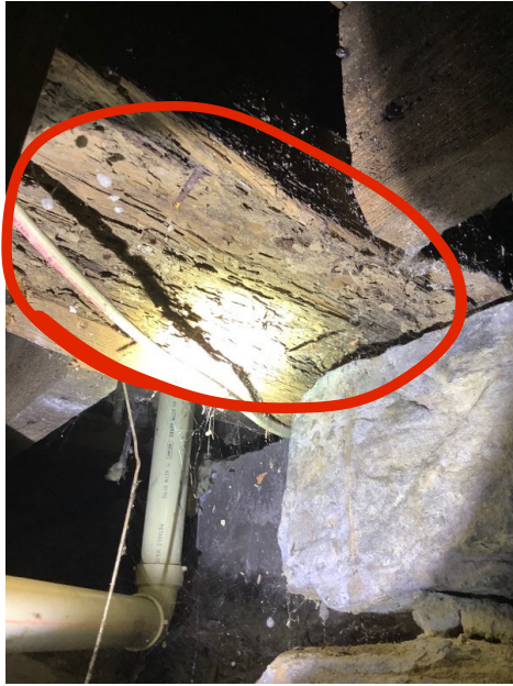
Both pictures crawl space opening beam over opening termite damage.
